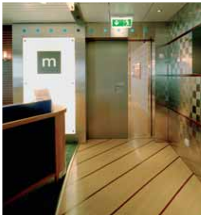
Internal sliding single fire door
