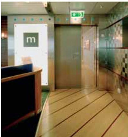
Internal sliding single fire door
